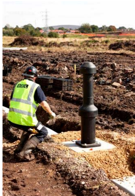
Combination bollards during installation on a virtual curtain gas migration barrier
