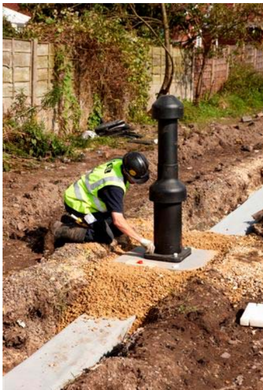
Combination bollards during installation on a virtual curtain gas migration barrier
